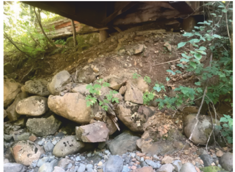
Left Bank Abutment when facing downstream
