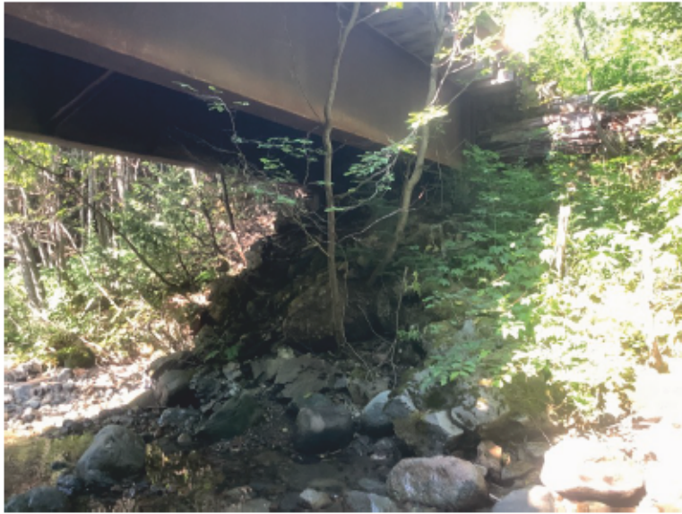
Right Bank Abutment when facing downstream
