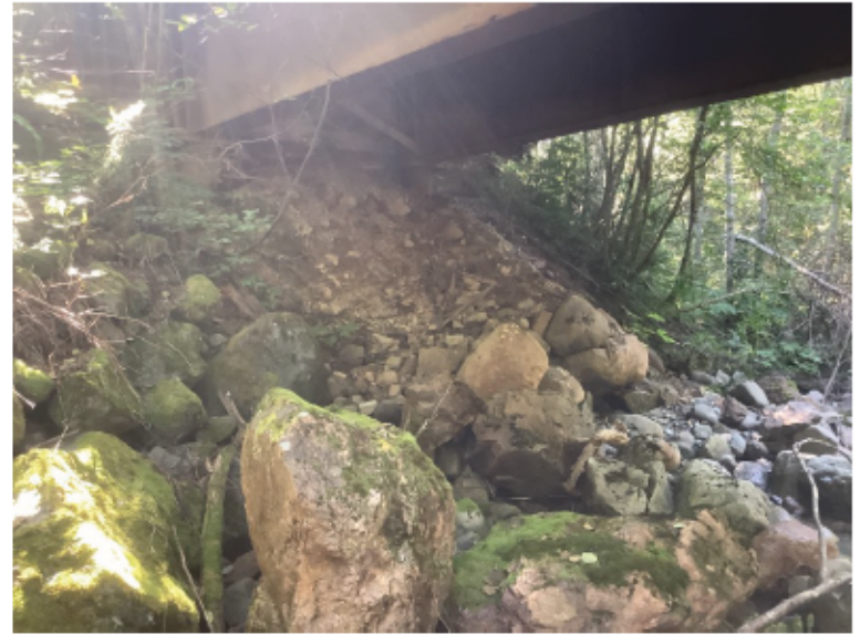
Left Bank Abutment when facing downstream
